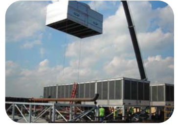
▲ The Grunau team installed rooftop cooling towers needed for Potawatomi Bingo Casino's new HVAC system.
